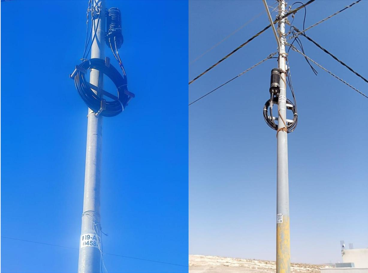
**Cross - Aerial Cable Storage Configuration for Angled Cables**
